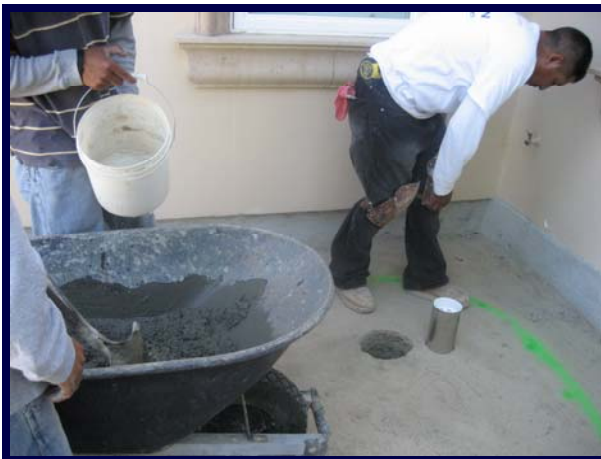
Dig out the hole for the cup.
