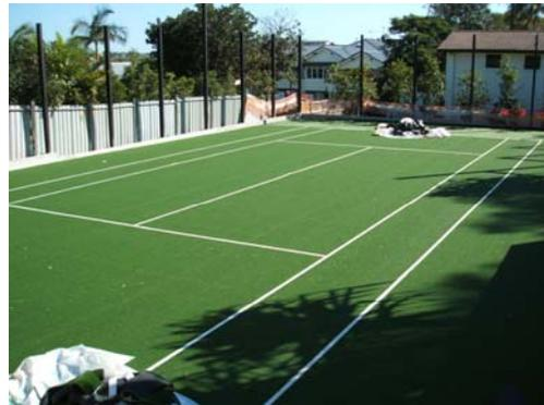
(usually about 20 minutes) this rolling process should be re-done to cement the bond. Subject to both the adhesive and the weather conditions no stress should be applied to this bond for a minimum of two hours. This process is repeated over the extent of the sport's area and left until adhesives are cured sufficiently to allow application of the sand infill.
