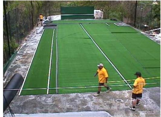
The combination of the yarn material used to produce the pile and mineral sand infill creates a sports surface with characteristics unlike most other tennis surfaces. Now twenty-five years from its introduction to the Australian market, it has found its place in many tennis clubs and on a majority of private courts around the country and is most popular for resort courts and with older players.
