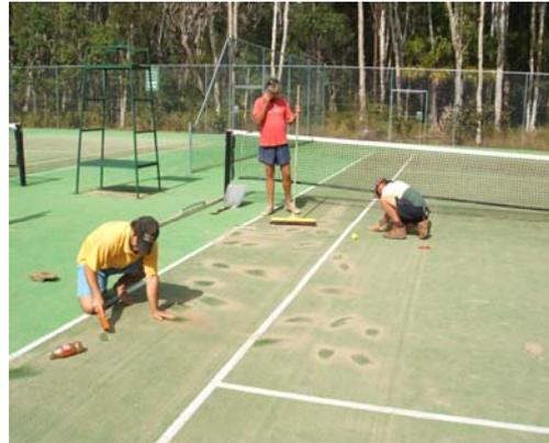
Environmental issues play a large part in the required maintenance of SFAG, with fallout from trees, algae growing in areas often shaded by trees, overland flow from poor drainage and general fallout from adjoining industry or the atmosphere. These elements affect hardcourts, driveways, the roof of your house and in fact most areas of the home, but are often not noticed on the textured surface of a SFAG court until they (the algae for instance) are well entrenched.
