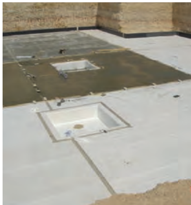
Protected Slab with exposed Water Stops
