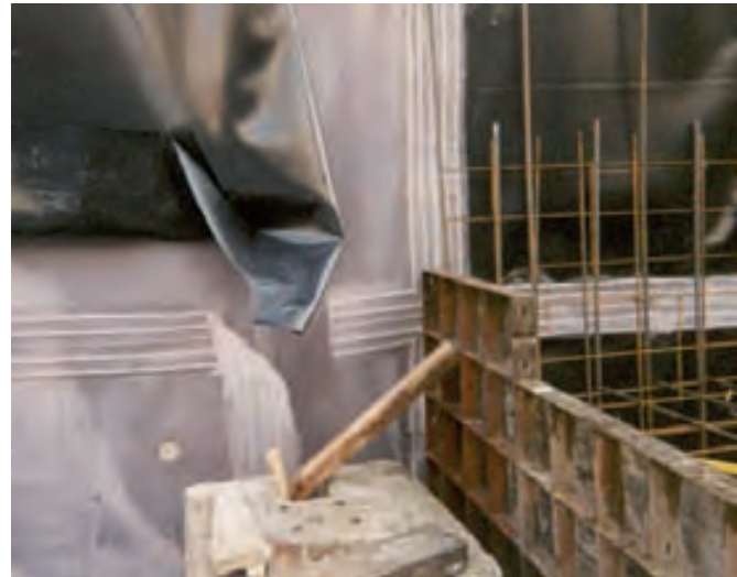
Execution of lining system with water stops
