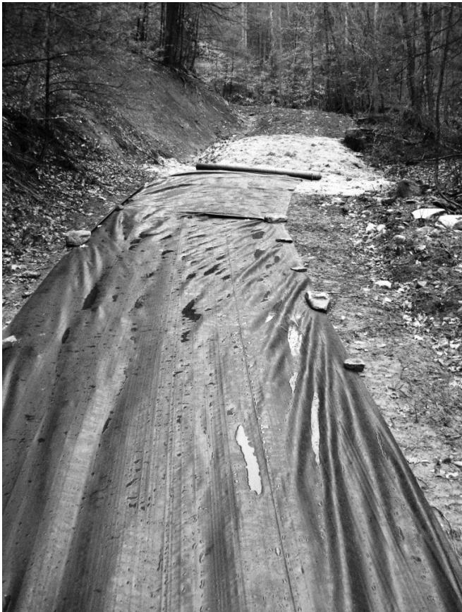
Photos of geotextile underlayment and stone aggregate applied atop a freshly-graded forest road on Rendezvous Mountain Educational State Forest in Wilkes County, NC. March 2008.
