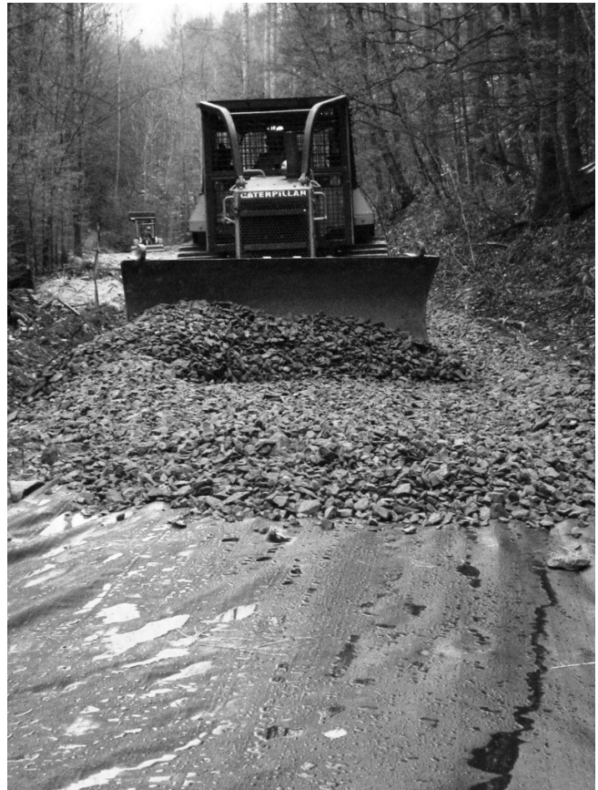
Photos of geotextile underlayment and stone aggregate applied atop a freshly-graded forest road on Rendezvous Mountain Educational State Forest in Wilkes County, NC. March 2008.
