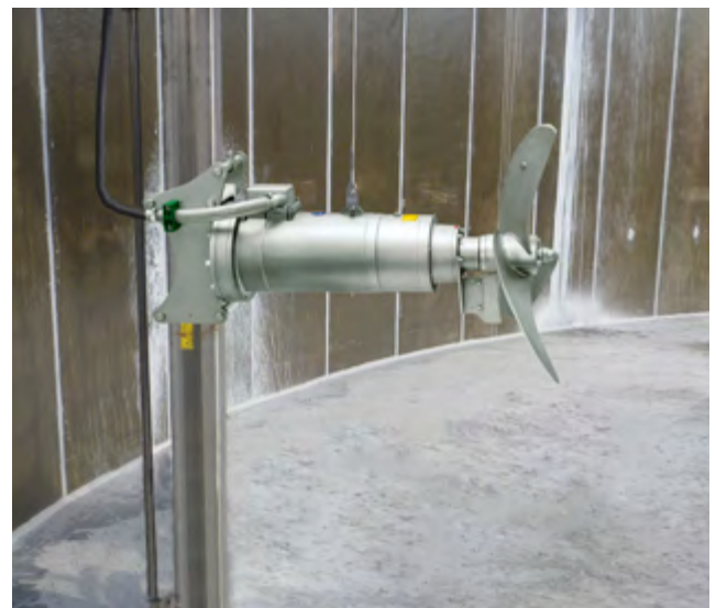
3A - Steel tank
