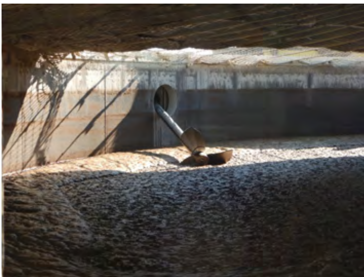
FTX - Concrete tank
