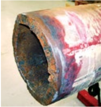
Hot torch cut before machining
